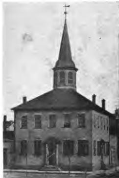
OLD COUNTY COURT HOUSE, LISBON
